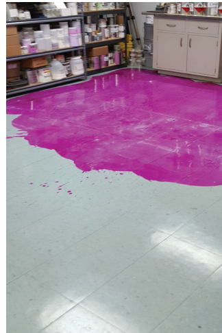
Floor being stripped.
